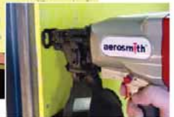
DensGlass® / Gypsum Sheathing to Steel
