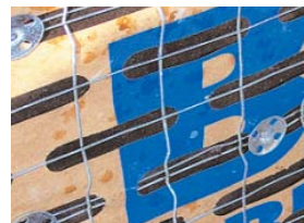
DensGlass® / Gypsum Sheathing to Steel
