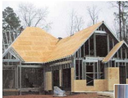
Plywood/OSB to Steel
